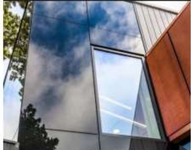
Aluminium windows adjacent glass cladding panels
