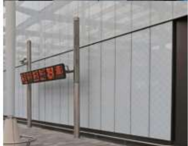
Glass cladding panels at Paddington Station/ Elizabeth Line
