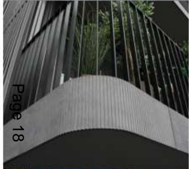
Metal balustrading adjacent GRC cladding panels
